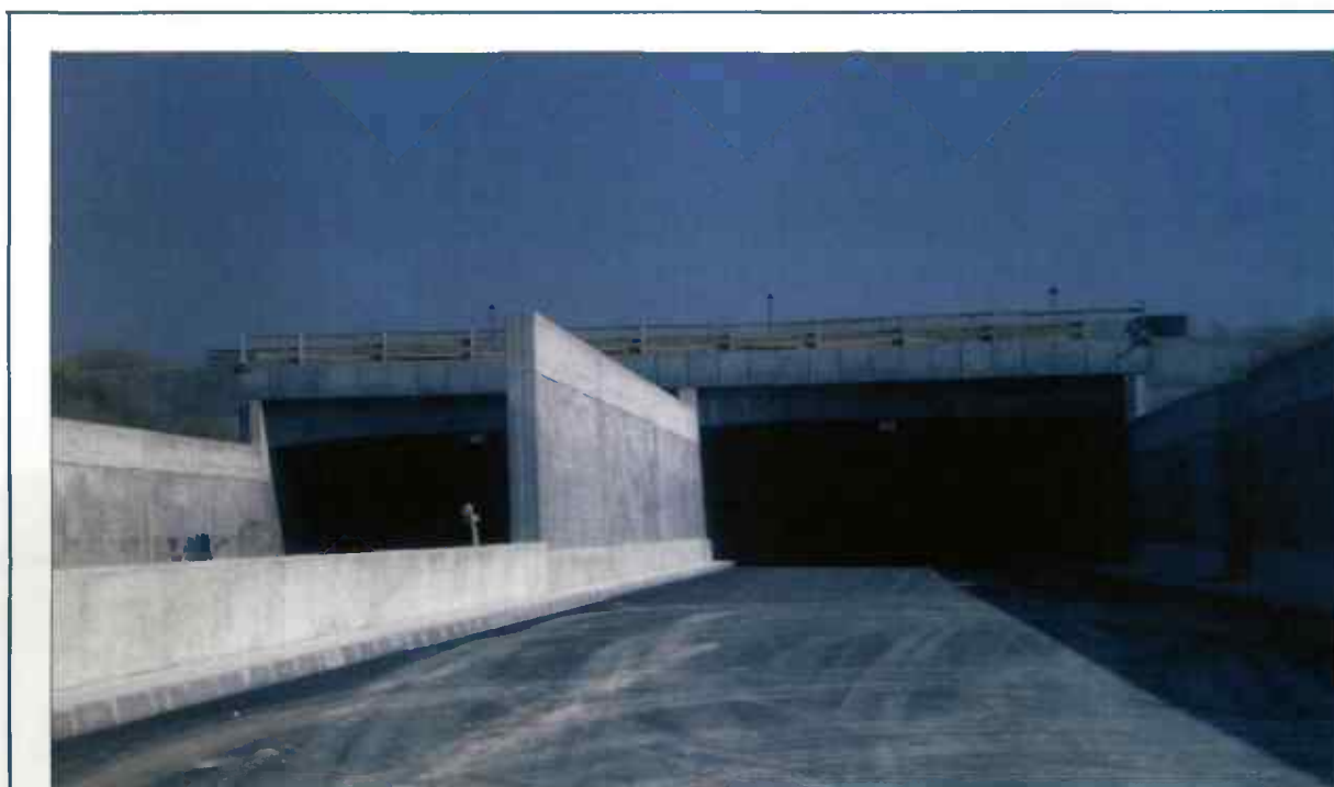
Figure 2.3 MUR ANTIRECYCLAGE
